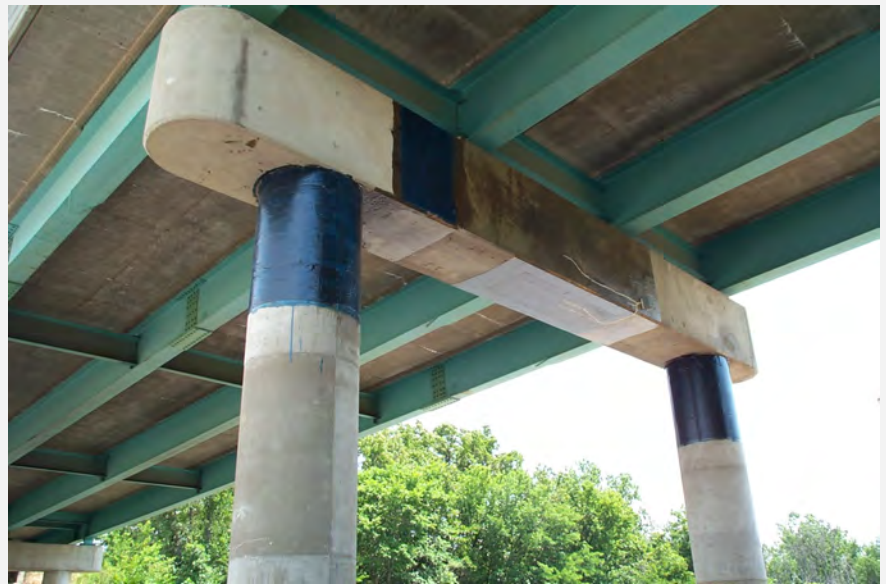
Fig. 8 Fiber optic sensors installed on the reconstructed pier cap of an I-44 Overpass. The crack sensors and the patch box are visible on the face and the delamination sensors are placed on the blue reinforcing sheet on the bottom.
