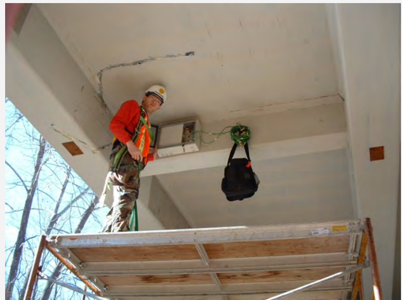
Fig. 9 Fiber optic sensors and patch box installed on the rehabilitated highway bridge. Sensors monitored both the bridge deck and girders.
